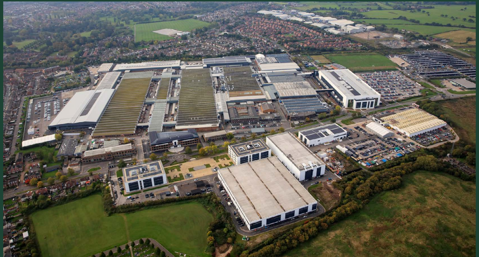
Bentley site in Crewe, UK
